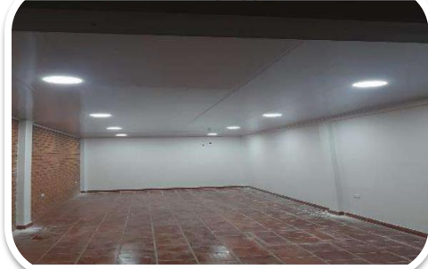
3.8.10 LAMPARA EMPOTRADA REDONDA LED 18 W
